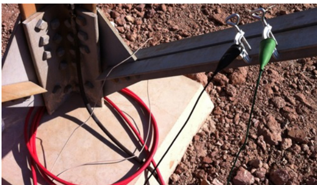
Output leads installed on a tower leg
