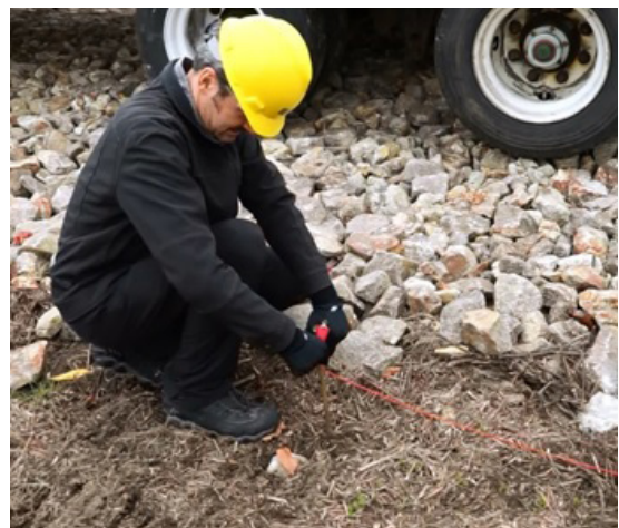
Installing an electrode
