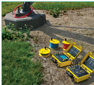
Flexible sensors measure leakage current and resistance on tower legs
